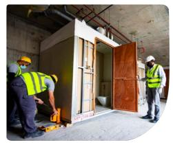
In some cases it may also be possible to use a specially designed lifting cage or cradle that is used to lift the pod to the desired level. The cage is then strapped to the building and the pod is wheeled out and into the building.
