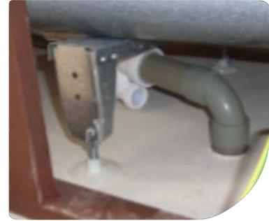
All drainage systems fitted within the pod are factory tested as part of our factory production quality assurance procedures. Test results for each pod are recorded and supplied with the pod as record and confirmation of testing procedure (see "Testing & Quality Control" for more details).
