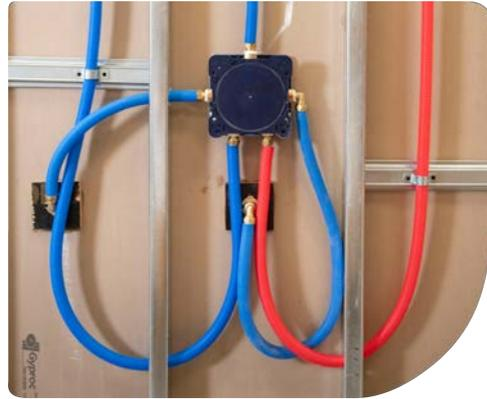
Pipework installations on every pod are rigorously tested as part of the factory production quality assurance procedures. Test results for each pod are recorded and supplied with the pod as record and confirmation of testing procedure (see “Testing & Quality Control” for more details).
