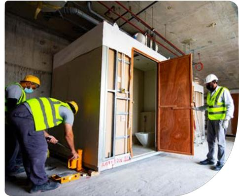
On low-rise projects and lower floors of multi-storey constructions it may also be possible for pods to be lifted to opening on intended installation floor by use of a fork-lift or telescopic handler.
